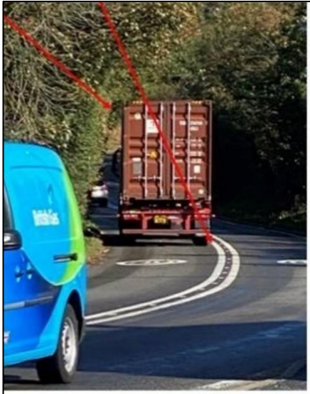
Plates 4 and 5: Standard width and length HGVs sit just within double white line system at Little Glemham
